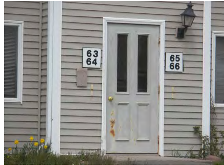
Common entry doors exhibit rust and impact damage
