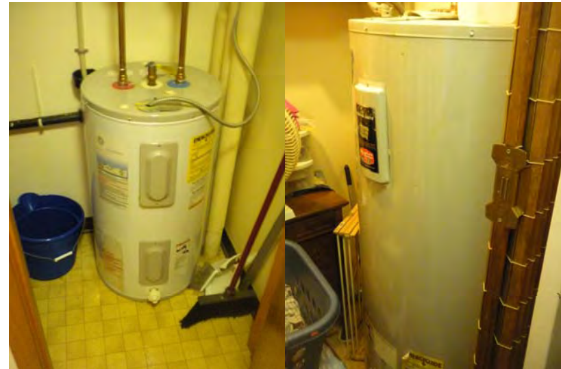
Typical unit level domestic hot water tank (left) and shared DHW tank (right)
