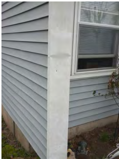
Siding and trim exhibit age related wear and damage
