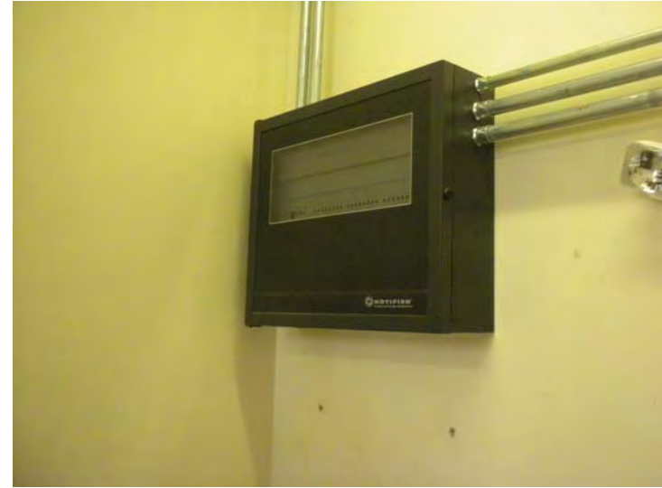
Example of the fire alarm control panel
