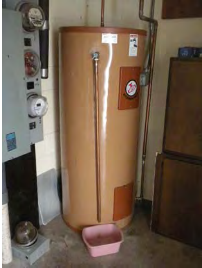
The laundry room domestic hot water tank
