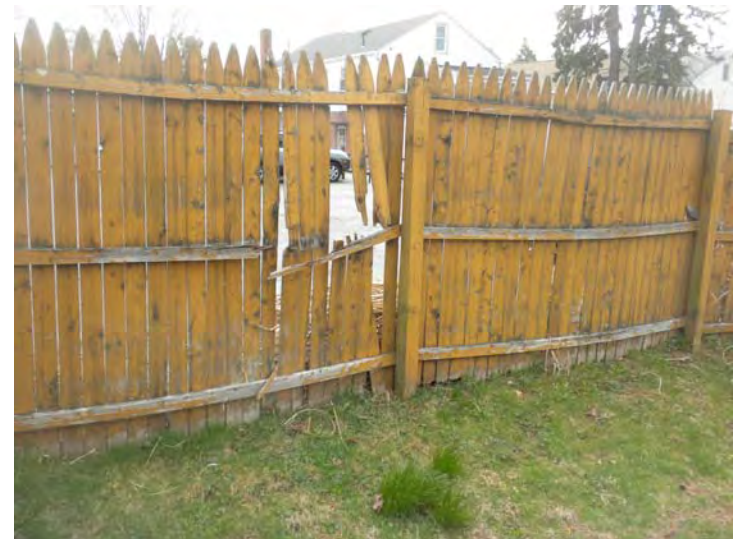
Damaged section of the wood picket fence
