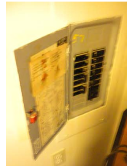
Example of a unit circuit breaker panel
